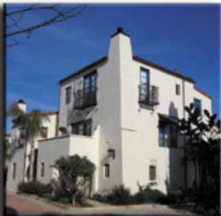
Townhouses & Condominiums: Villa Del Mar (40 Units)
