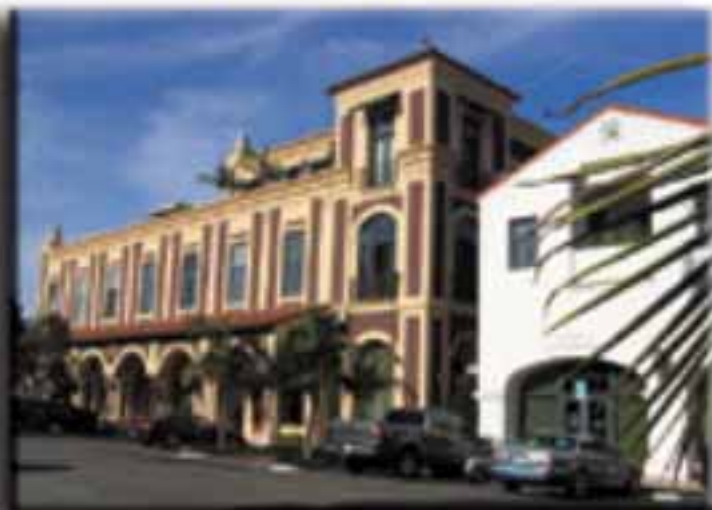
Commercial/Residential Mixed Use: Chapella Lofts
